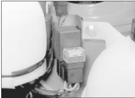
3.7a Headlamp washer relay and fuse
